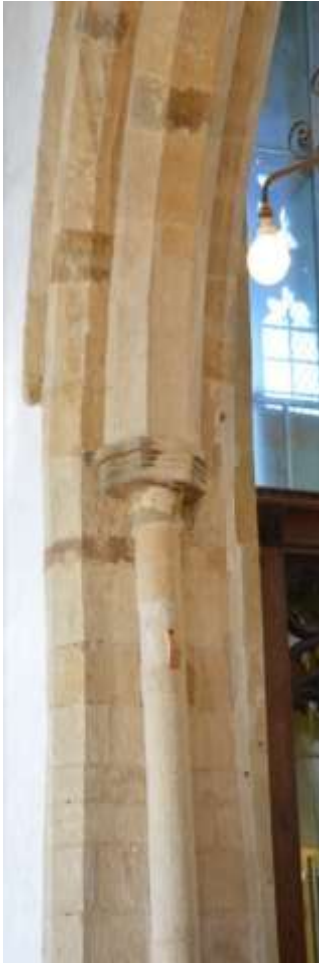
The single pillar, showing the style of the earlier design of the southern range of arches.
