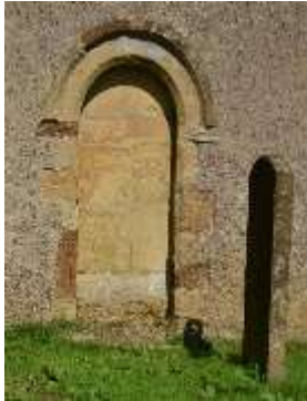
Arched doorway in north wall of chancel © David McGill
