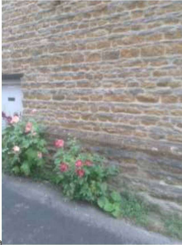
An example of alternating courses of ironstone and oolitic limestone in Queen Street.
